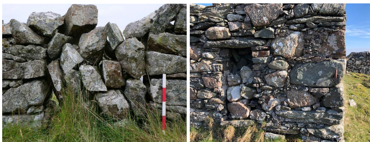
Figure 6: One of the crudely block entrances to Building 4 (left); Mortared joints and roughly dressed quoins of Building 5 (right). (Photographs: Trevor Pearson & Elaine Jamieson)
